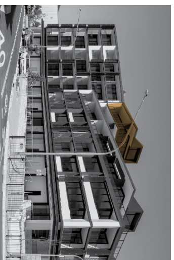
Fig. 7.5.23 Attic level setback Source: Union Bahrain, Turner, 2019
